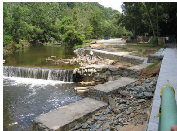
4. The long narrow wall to the right of the person standing above the dam is the fish ladder containing the baffles that allow the fish to climb and rest to get above the dam.
