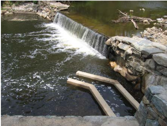
1. At the lower end of the channel, fish feel the flow of water and swim into the fish ladder.
