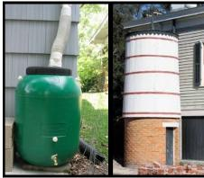
These tools are often used to capture rainwater runoff from the roof of a building. The water can be held for a period of time and then reused to water gardens during a dry period or for other purposes. However, once a barrel or cistern is full, water will continue to runoff as before.
