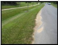
Filter strips are areas used to slow down the flow of water impervious surfaces. These strips can also act as a cleaning device as the water runs through the vegetation and even infiltrates the ground. They provide a simple solution but may not be able to manage extreme storm events and are highly dependent on having low soil compaction.
