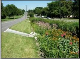
A bioswale is very similar to a rain garden. However, they are frequently designed to capture and filter larger volumes of water. To do so requires more deliberate engineering of soils and layers. The plants in a bioswale will be able to withstand different levels of water once established. These areas are usually located near impervious surfaces.
