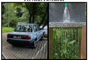
Pervious pavement exists in many forms but is mostly used to address the rate of flow during a rain event. To be considered pervious, the surface must allow water to percolate through the top layer. In some forms, this allows water to infiltrate to groundwater systems. A general outcome is that runoff is slowed and possibly minimized.
