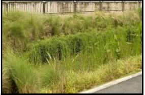
Rain gardens, also called Bioretention, usually consist of a small depression to collect water and improve water quality. These areas are vegetated with specially selected native plants that are native to the area and can adapt to varying conditions from dry to flooded. Soil that is too compacted will need to be amended before planting a rain garden in order to improve infiltration.
