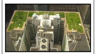
A green roof makes use of an impervious surface as a base for vegetation. The vegetation can then work to absorb stormwater, reducing the rate and amount of runoff from a building during a rainfall event. If constructed properly, a green roof can also improve the quality of runoff water. However, it may take five or more years to reach an efficient level of pollutant removal.
