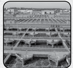
photo: Courtesy of DC Water.
